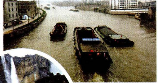
Beijing-Hangzhou Grand Canal
