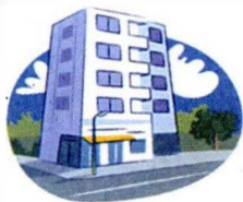
1 a block of flats
